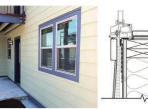
Earth Advantage is a certification that boasts 10% better than code in overall energy performance. From the wall section on the left, you can see that the Earth Advantage wall is similar to conventional light frame wood construction with insulation between studs.
